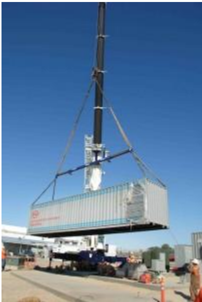
Crane Placing Battery Storage System at Santa Rita Jail
