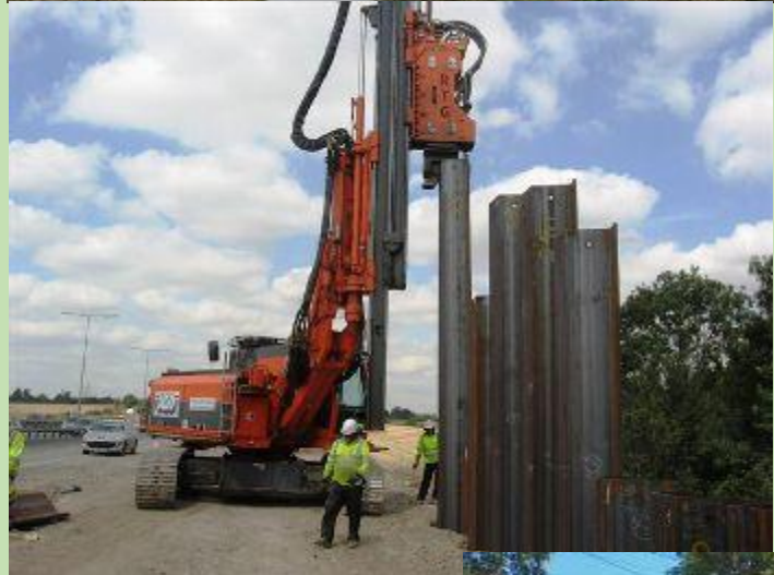
Hydraulic Press Machinery to Install Steel Sheet Piles for Channel Walls
