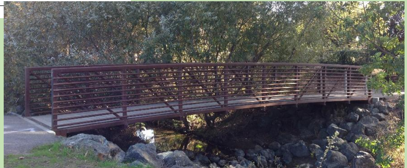
Example of Single Span Steel Bridge Proposed for new Gomes Park Bridge
