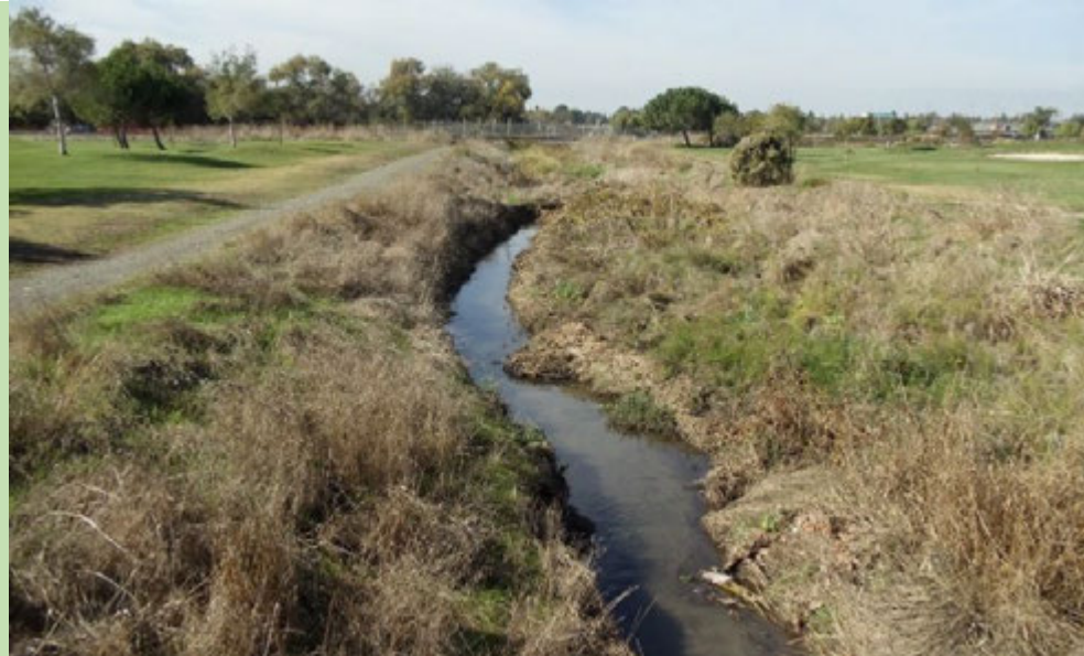
Looking downstream from Golf Course Bridge
