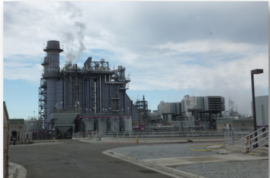
Russell City Energy Center
