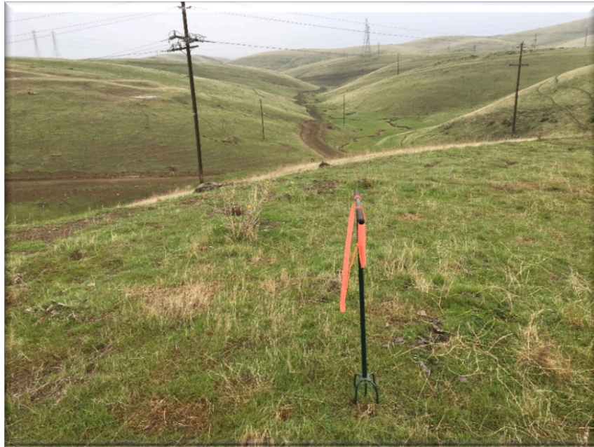
Plate 7. Example of decommissioned above-ground distribution lines that would be removed as part of the project.
