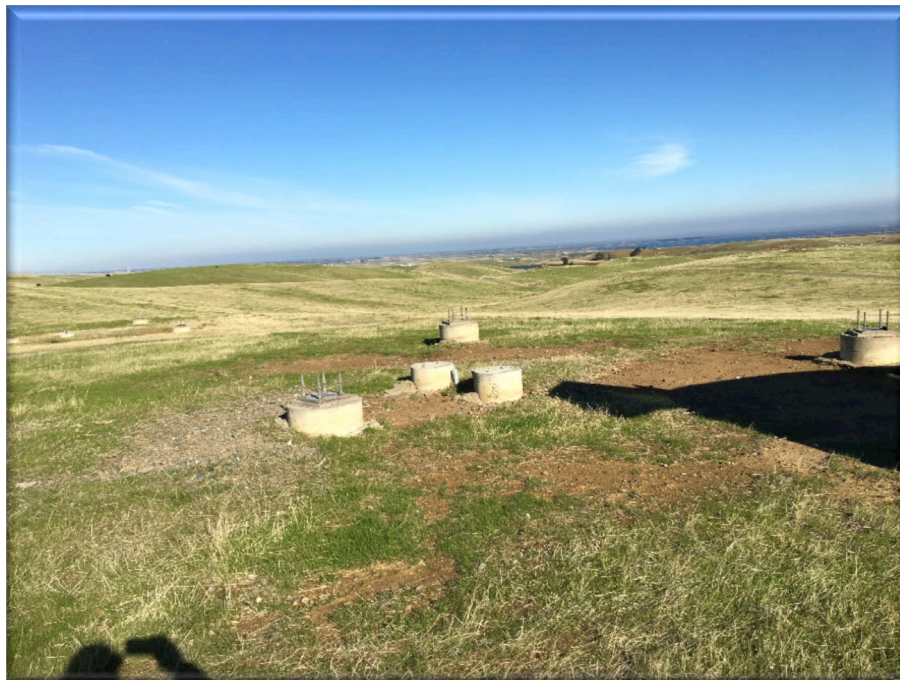
Plate 6. Example of concrete footings remaining following removal of decommissioned old-generation turbine string.
