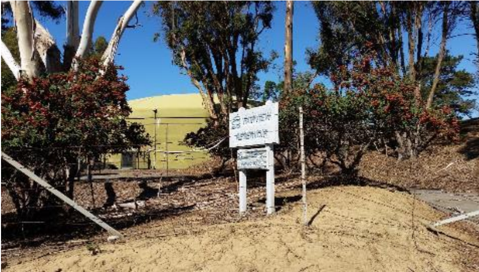
EBMUD water tank near Fairview Avenue
