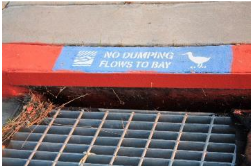
Stenciled storm drain along Maud Avenue
