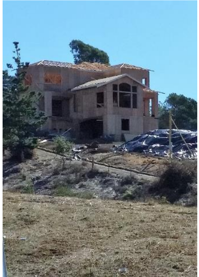
Hillside grading at a new Fairview home
