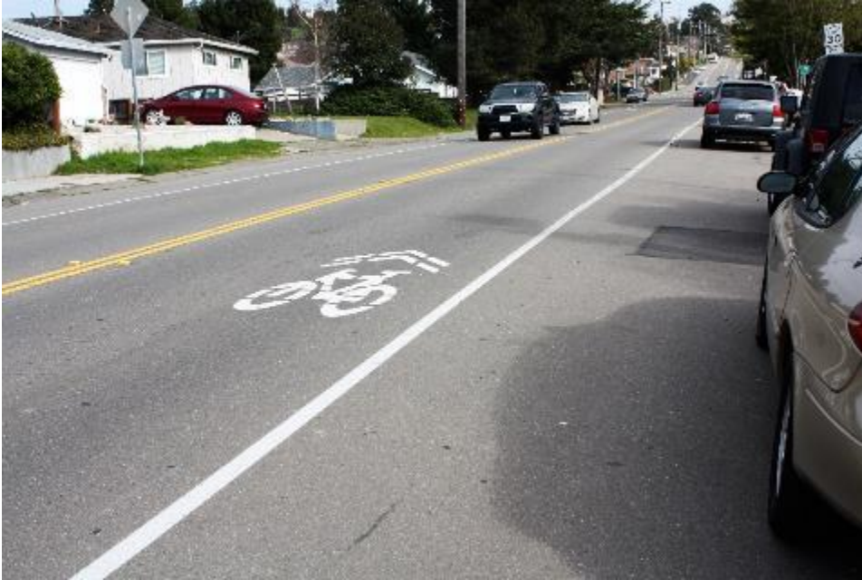
Sharrow (shared bicycle and vehicle lane) on D Street
