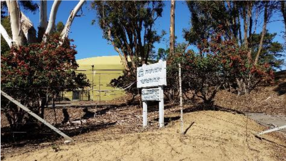
EBMUD water tank near Fairview Avenue
