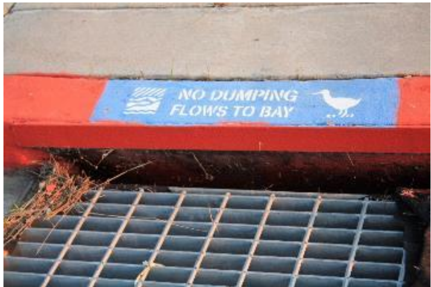
Stenciled storm drain along Maud Avenue
