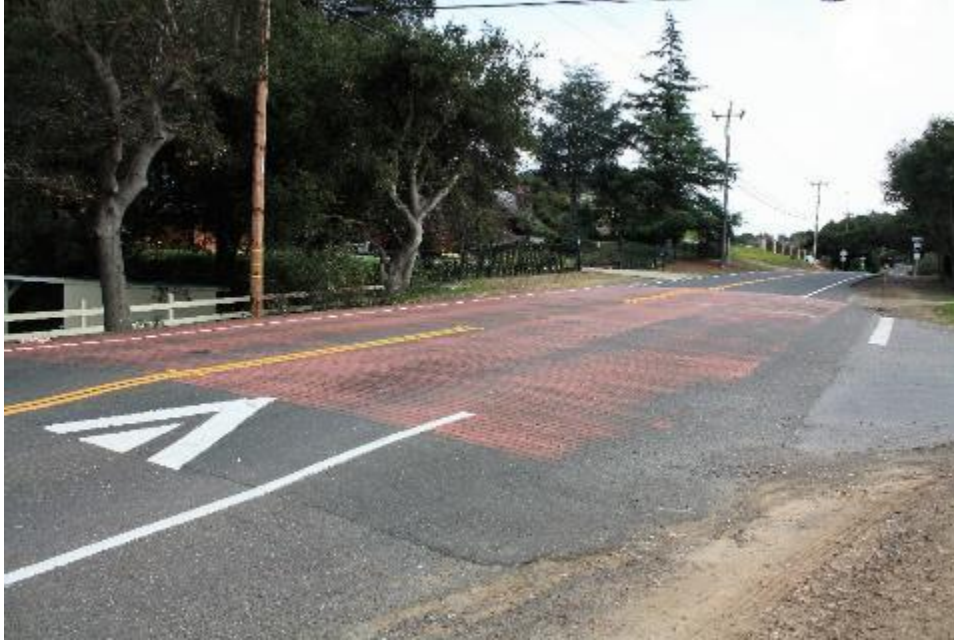
Speed table at Amyx Court and Fairview Avenue
