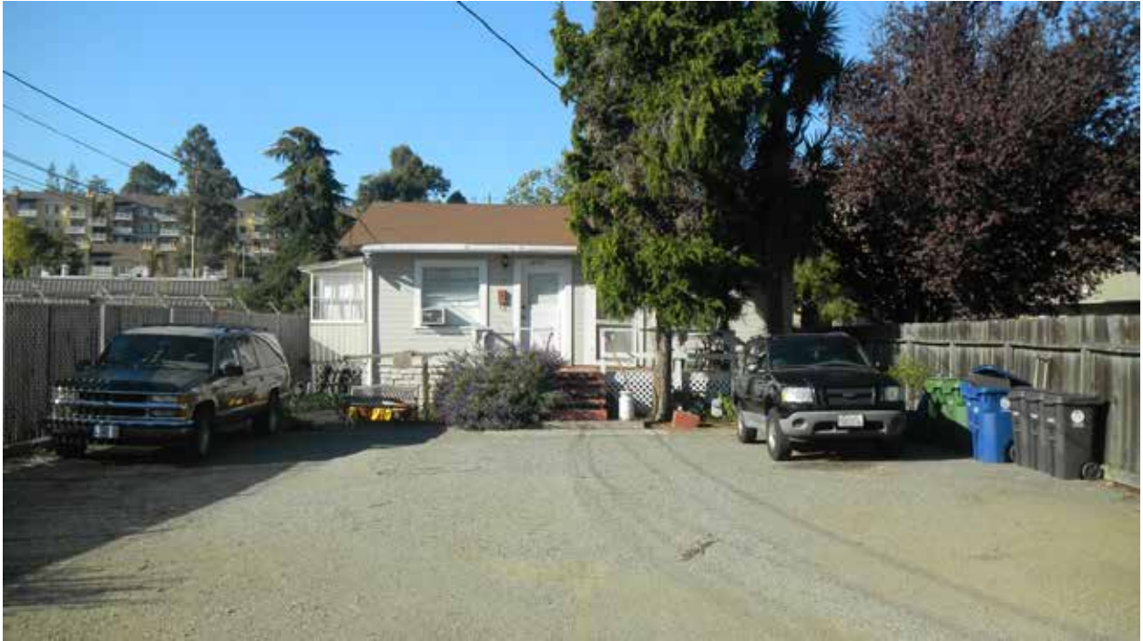
Fig.7 – 20785 Baker Rd. – Front (east) of front cottage (looking west)
