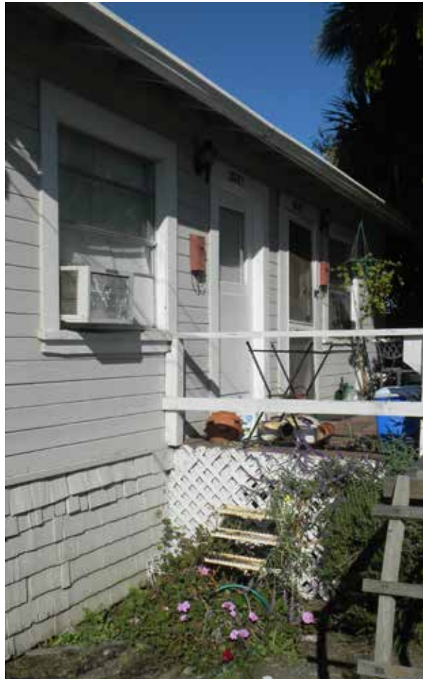
Fig.8 – 20785 Baker Rd. – Front of front cottage (looking northwest)
