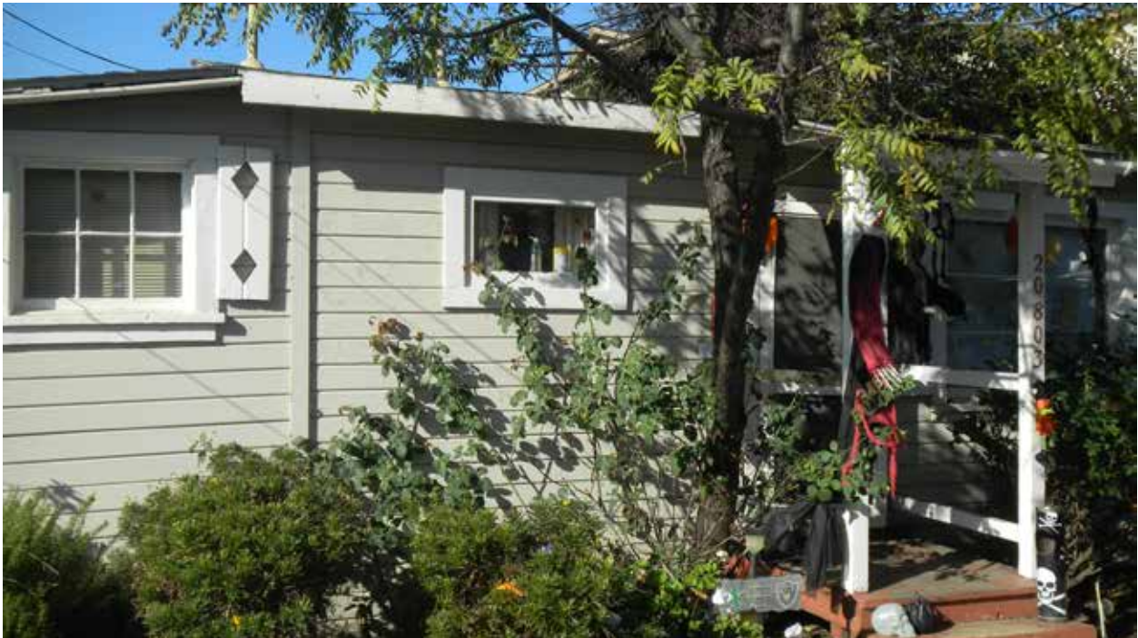
Fig.13 – 20785 Baker Rd. – Front of rear cottage (looking west)
