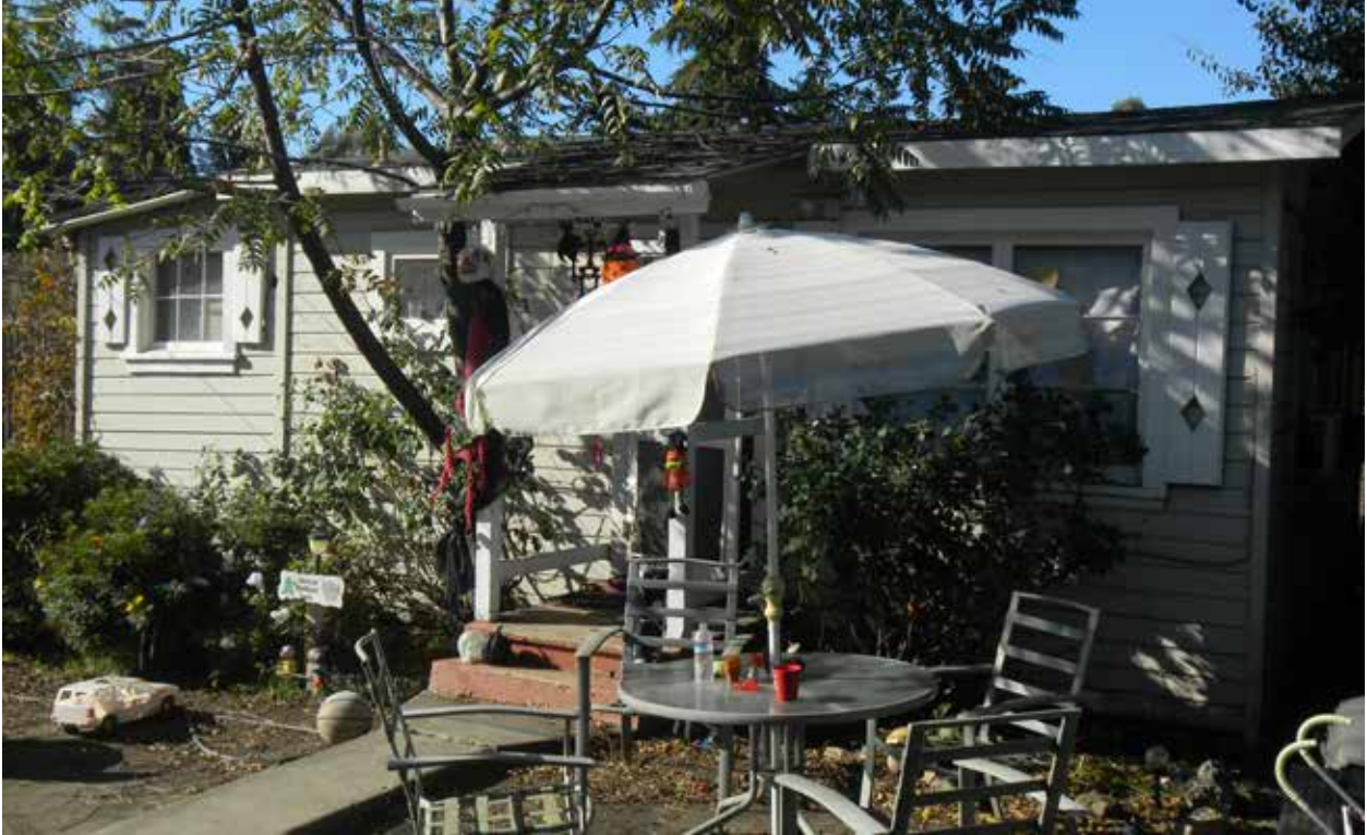
Fig.12 – 20785 Baker Rd. – Front of rear cottage (looking west)
