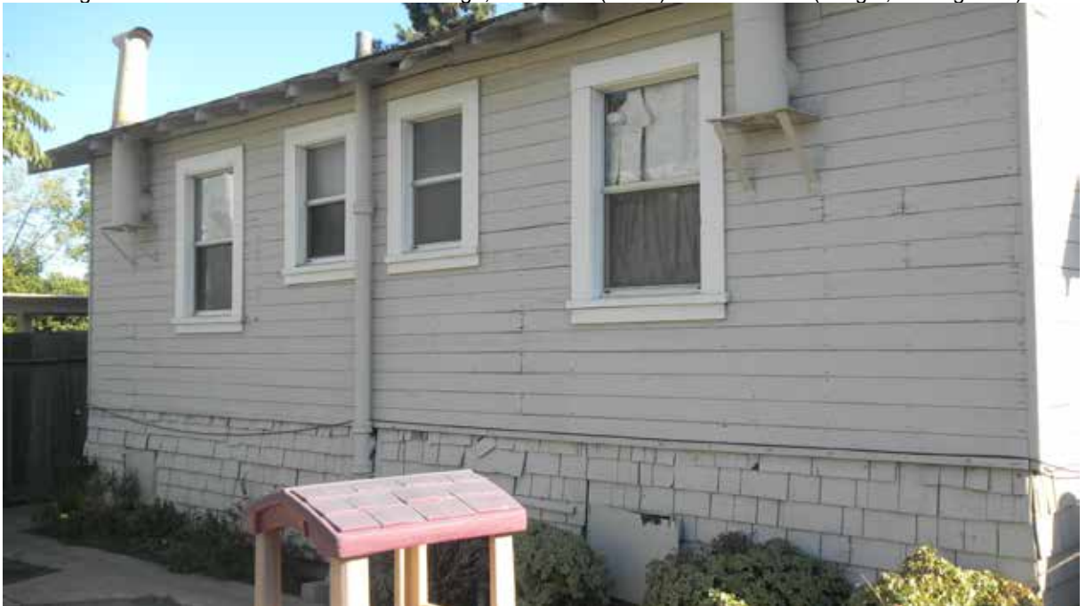
Fig.11 – 20785 Baker Rd. – Rear of front cottage (looking northeast)
