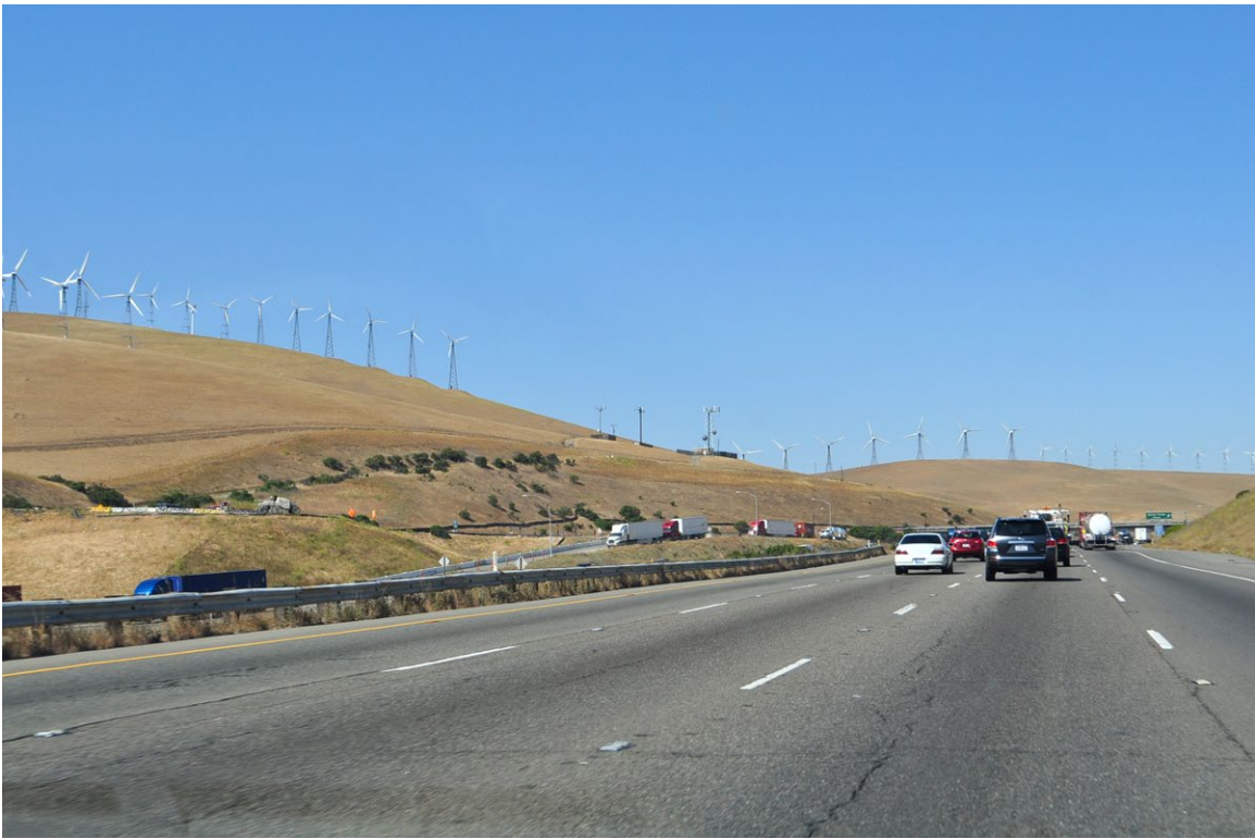
2. From westbound I-580 looking southwest.
