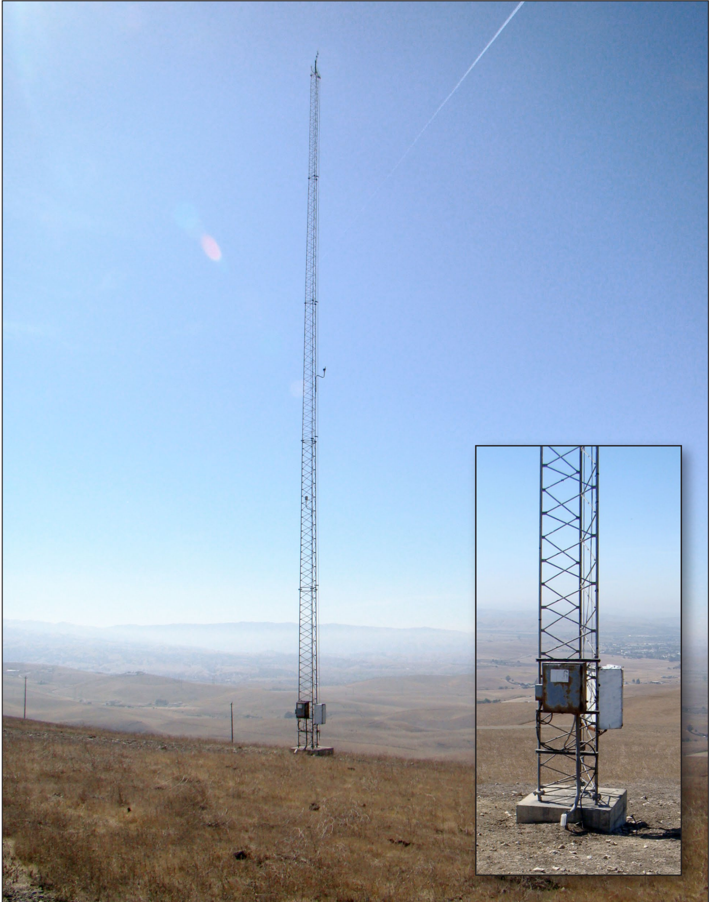
Figure 2-6 Free-Standing Permanent Meteorological Tower
