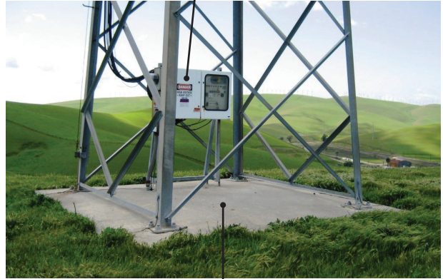
Spread Footing Foundation
