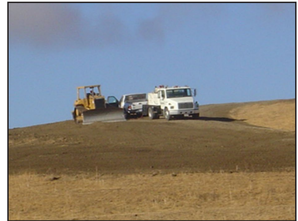
Graded area is ready for seeding
