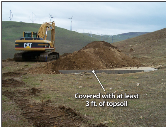
Foundation location on high slope area
