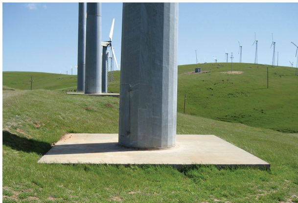
Spread Footing Foundation for Tubular Tower (Down Tower Cabinet inside Tower)
