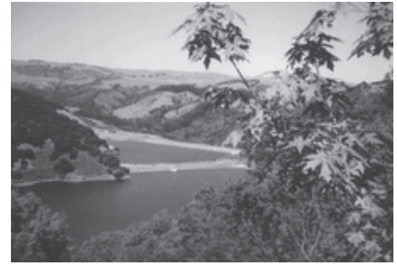
EBMUD has replaced the original dam at Upper San Leandro Reservoir.
