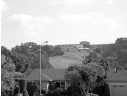
Castro Valley is located in an area with steep topography that is very near the Hayward Fault, which creates risks of ground shaking, liquefaction, and landslides.
