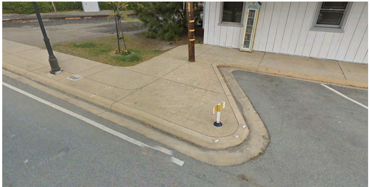
Looking Northwest at existing Area 6 sidewalk
