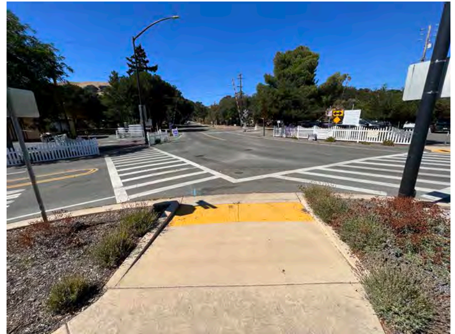
Looking North at the intersection of Main Street and Kilkare Rd
