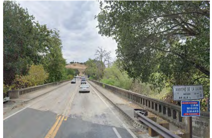
Looking East across the bridge
