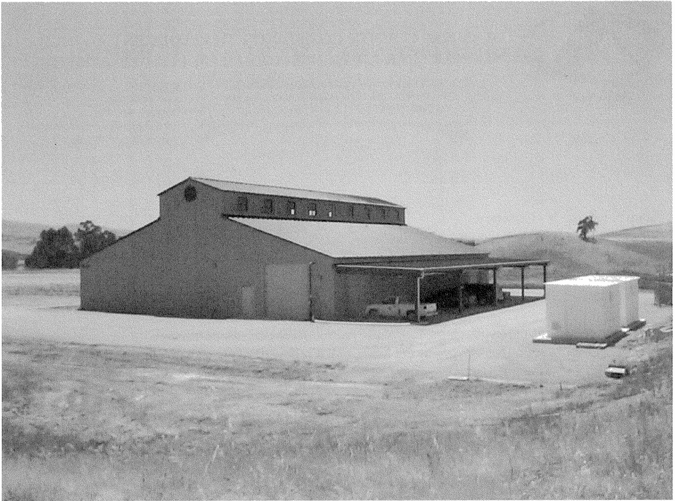
Construction of the new East County field office for the Alameda County Department of Agriculture/Weights and Measures was completed in May 2001. The office is located at 3575 Greenville Rd. in Livermore.
